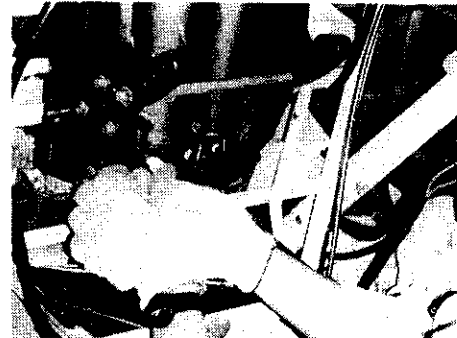
(Install the seal tape and the flare adaptor)
