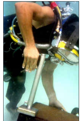
Figure 1: Diver using ramset
