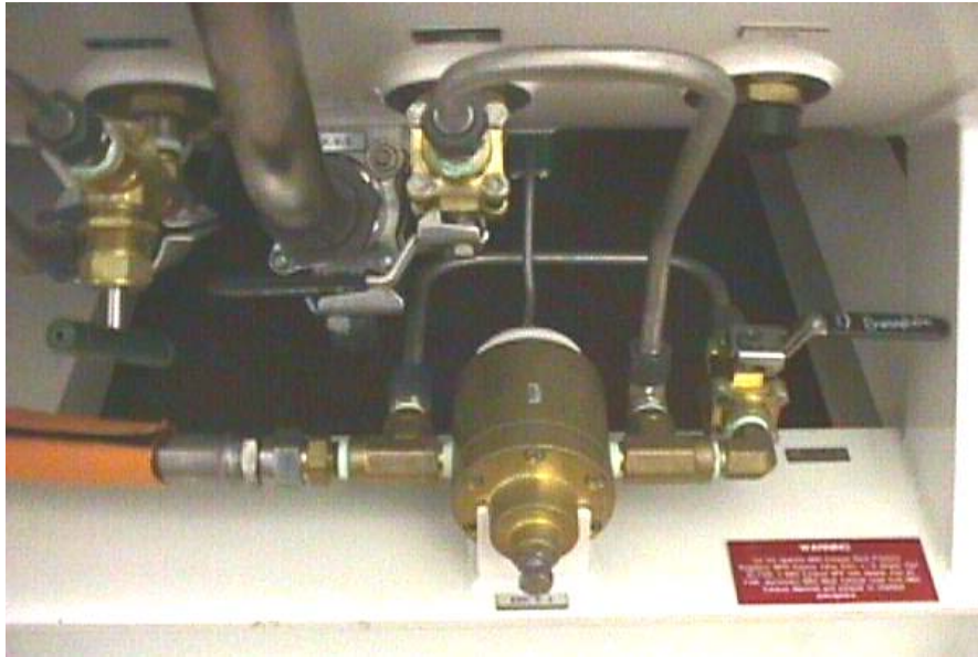
Figure 3-20. BIBS Exhaust Back Pressure Regulator
